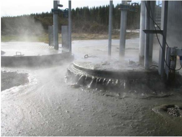
**Fig. 2** Foam overflow from the reactor of Lemvig biogas plant
